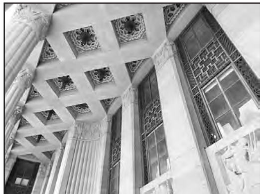
Detail of Buffalo City Hall.
