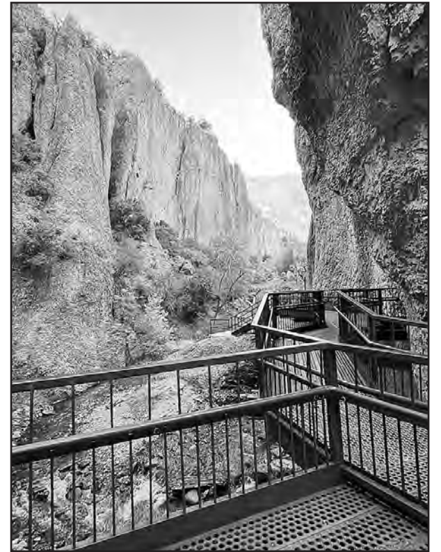
Catwalks near Glenwood, New Mexico.
